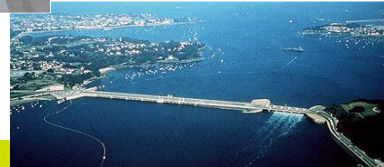
Tidal Power Station, La Rance, Brittany, France
