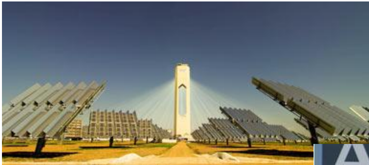
The world's largest solar power energy plant, Sanlucar la Mayor, Spain
